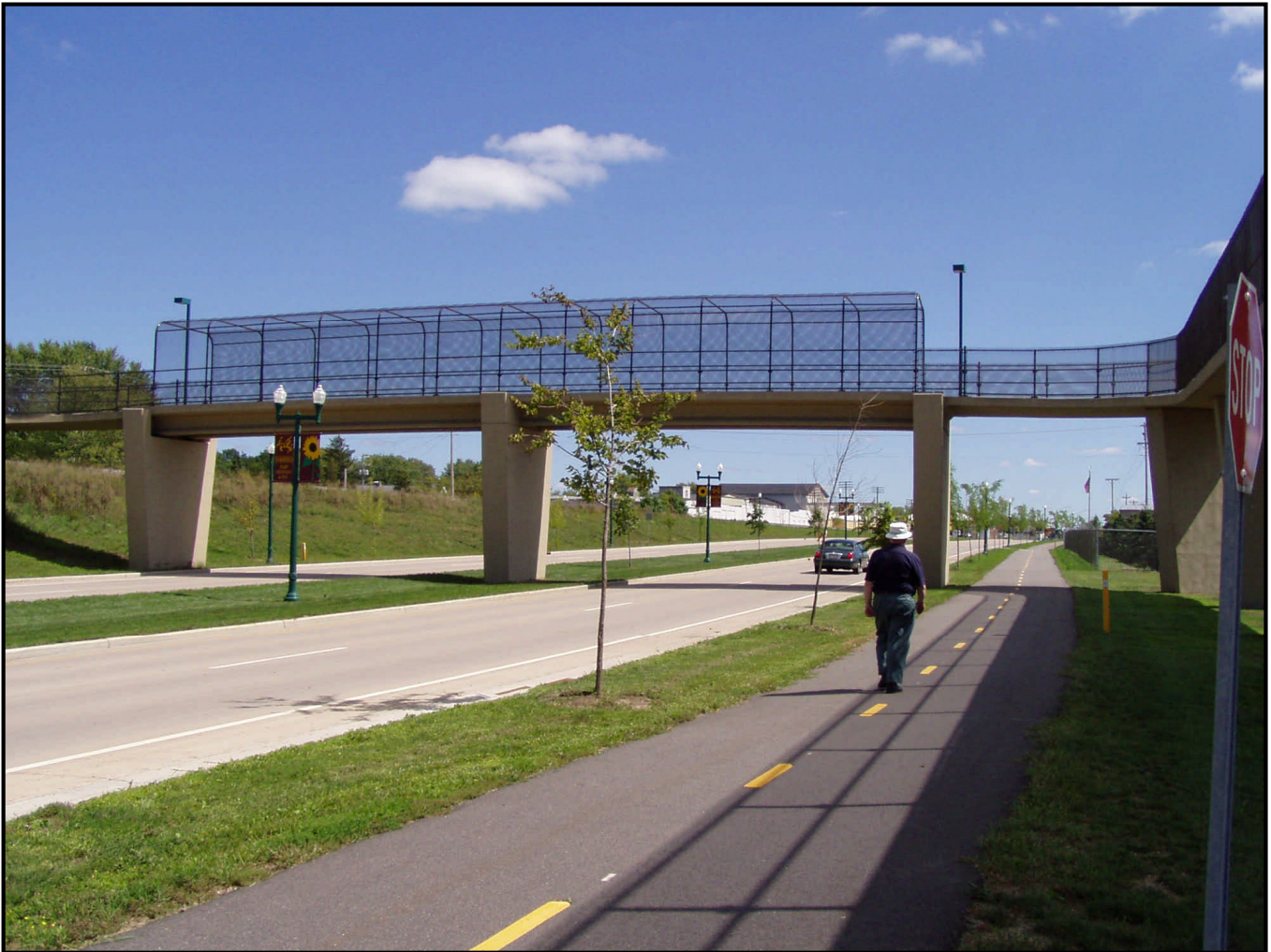
Veterans Parkway Pedestrian Bridge, Marshfield
